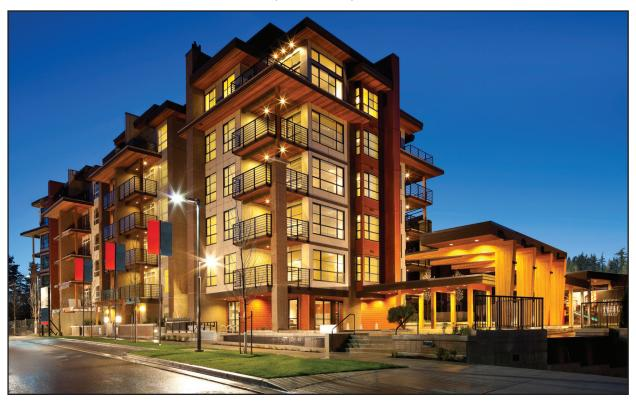
"The dynamic entrance canopy uses cleanly detailed glulam structural beams and striking wood soffits in this unified six-storey wood designed residential building."
