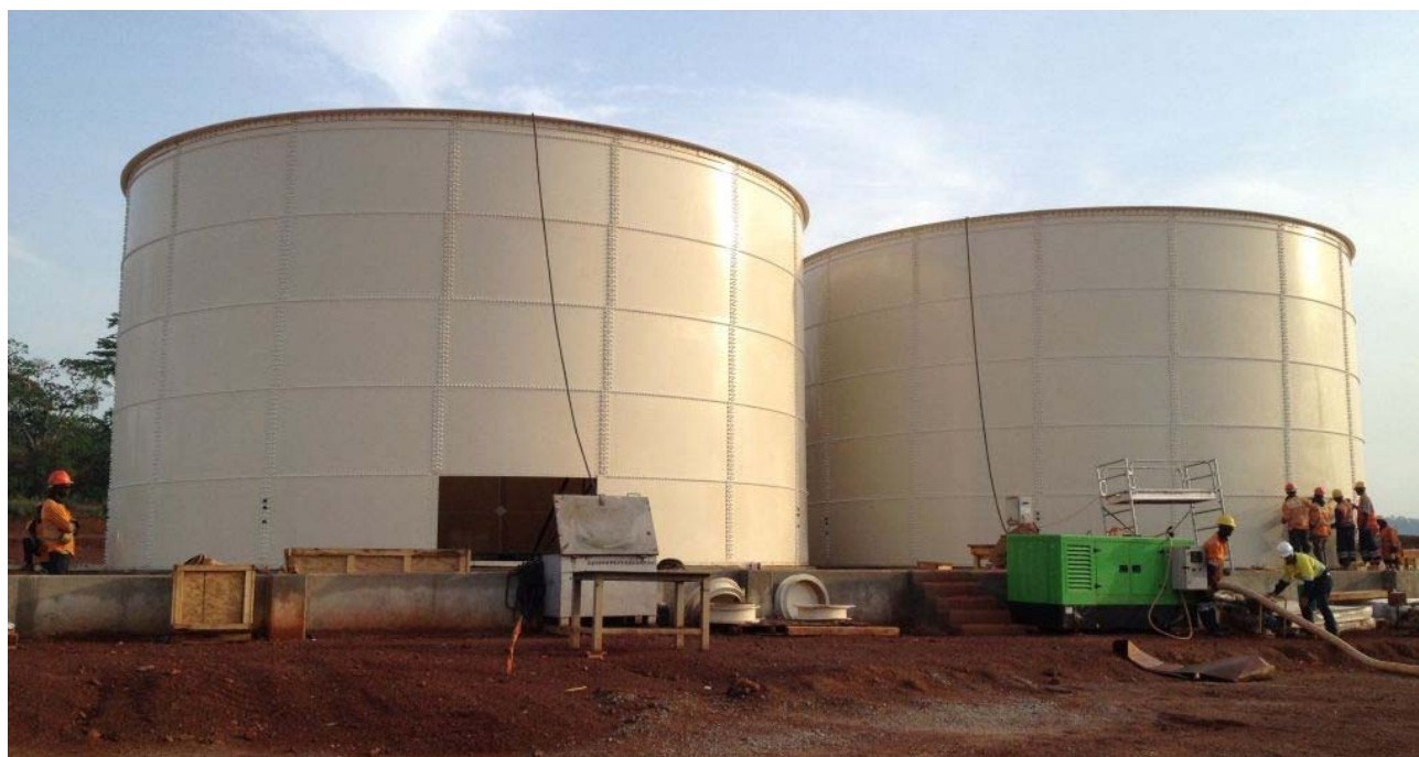
Figure 4: CIL Tanks March 2013
