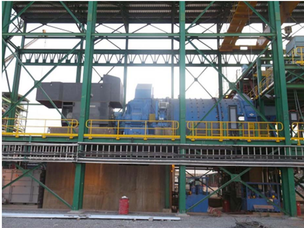
Figure 3: Tabakoto mill expansion
