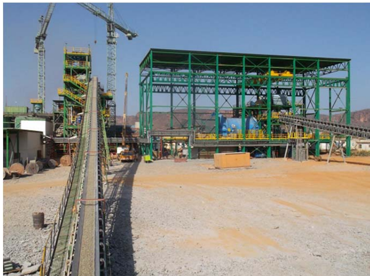
Figure 3: Tabakoto mill expansion
