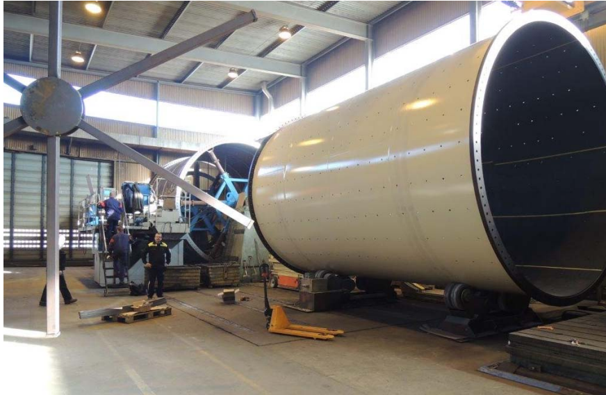
Figure 7: SAG and Ball Mill shells under construction
