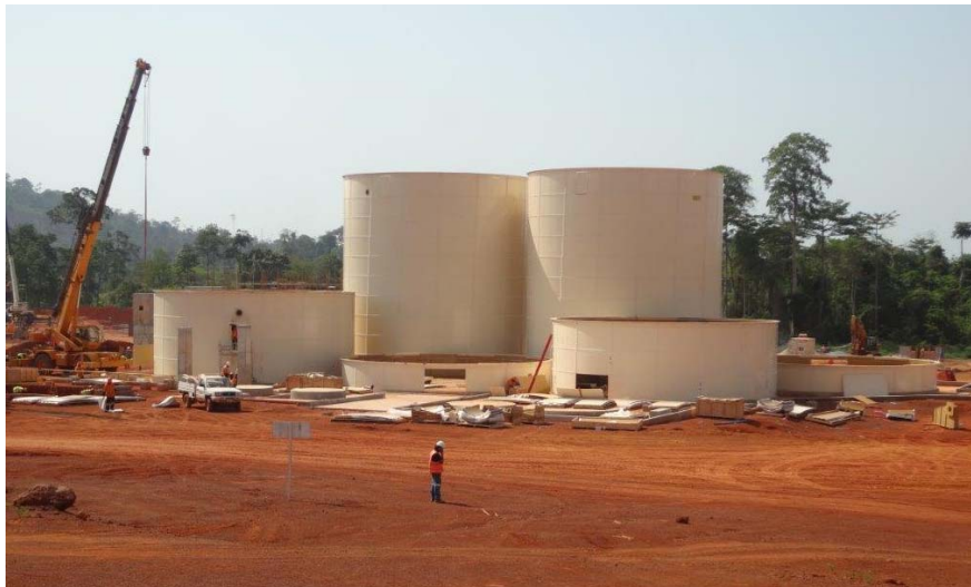
Figure 6: CIL Tanks March 2013
